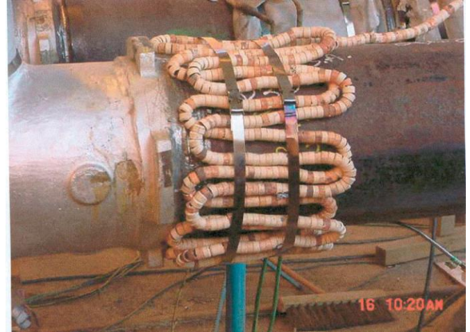
Detail the positioning of the resistance
