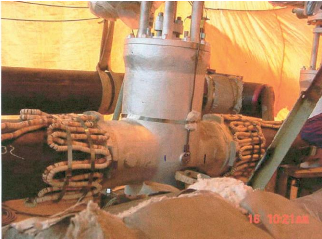
Valve body with resistance positioned correctly only in the regions of the bevels
