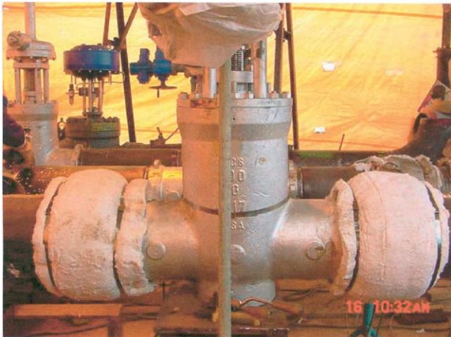
Valve body with mounted and isolated Resistance heat ready to start the heat treatment the welded joints.
