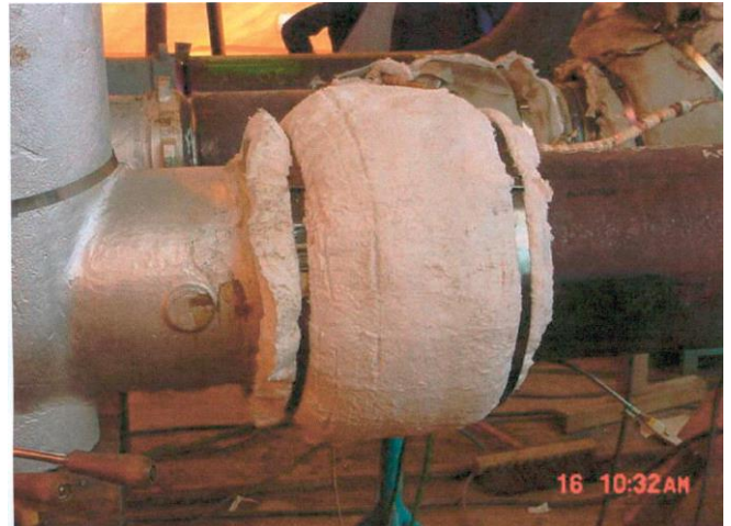
Detail of thermal insulation resistances
